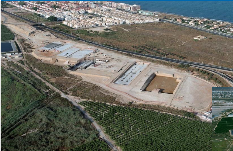
Starting of the works in February 2007
