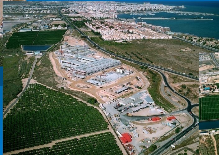
Current state of the works
