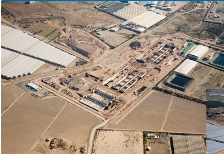
Starting of the works in June 2007
