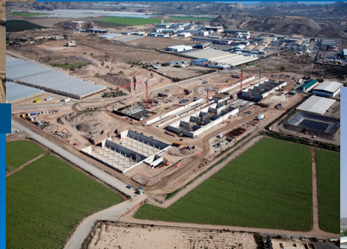
Current situation of the works
